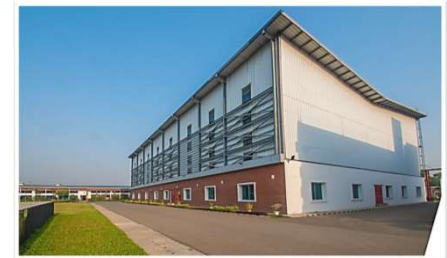
Central Warehouse(Full View)
