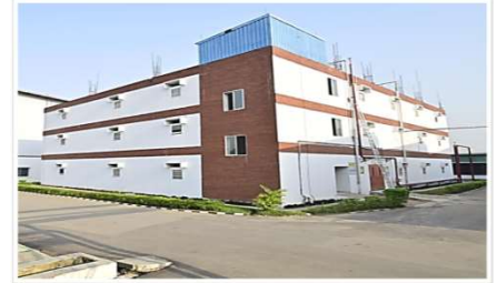
Chemical Store(Full View)
